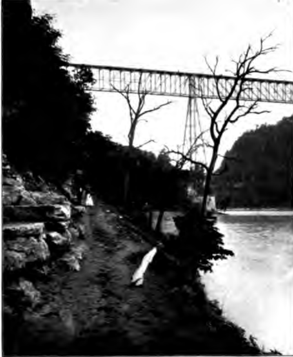
PATH ALONG THE CLIFFS. HIGH BRIDGE.
